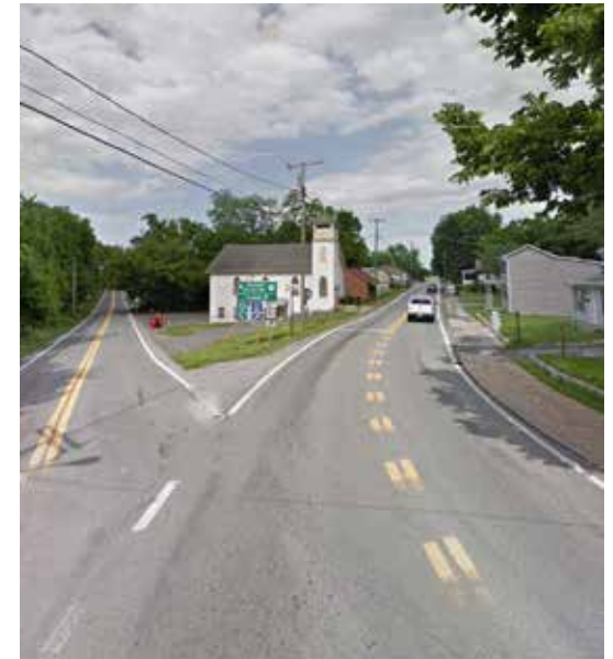
(Above, right) The triangular intersection of WV-51 and CR-13 has a crash rate 2.6 times higher than the state average (based on traffic activity for 2015-2019). Looking west into the intersection, it's easy to see that the transition from the rectangular grid of the downtown streets into the tangle of turning options, driveways, and unusual sightlines can pose challenges for motorists, bicyclists, and pedestrians.
