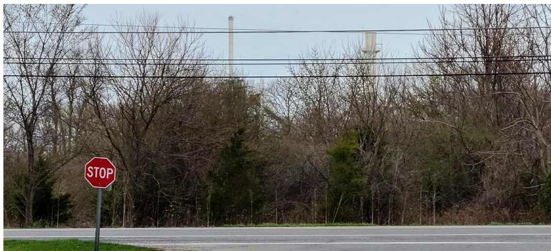
The Rockwool mineral wool factory, scheduled to begin production this spring, is visible across the road in front of North Jefferson Elementary School.
