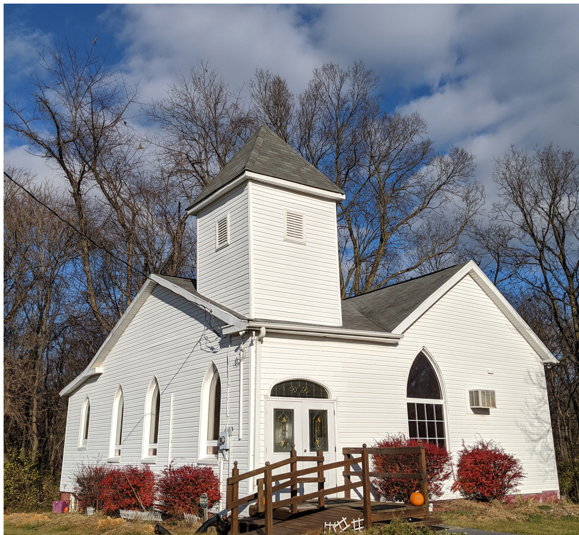
The historic structure of St. Paul Baptist Church continues to serve an active congregation.
