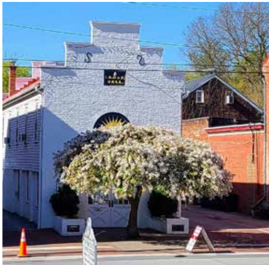
The Jefferson County CVB is collaborating with the Town of Shepherdstown to rehabilitate the historic Market House in downtown for use as a welcome center.
