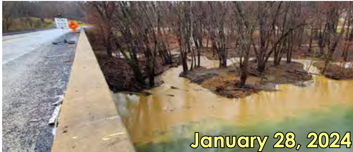
Image above: The sediment-filled Evitts Run flows into the Shenandoah River just below the Bloomery Bridge (Route 115), downstream of the Blake solar facility. Image next page: Sediment discharge flows directly from the Blake solar facility. According to US EPA studies, excessive sediment runoff can alter river habitats, reduce water oxygen levels, and trigger declines in aquatic animal populations. Text box next page: Excerpt from violation notice issued by WV Department of Environmental Protection to the Blake Project in July 2023. Visit ObserverWV.com/tracking-solar for more images and video links.
